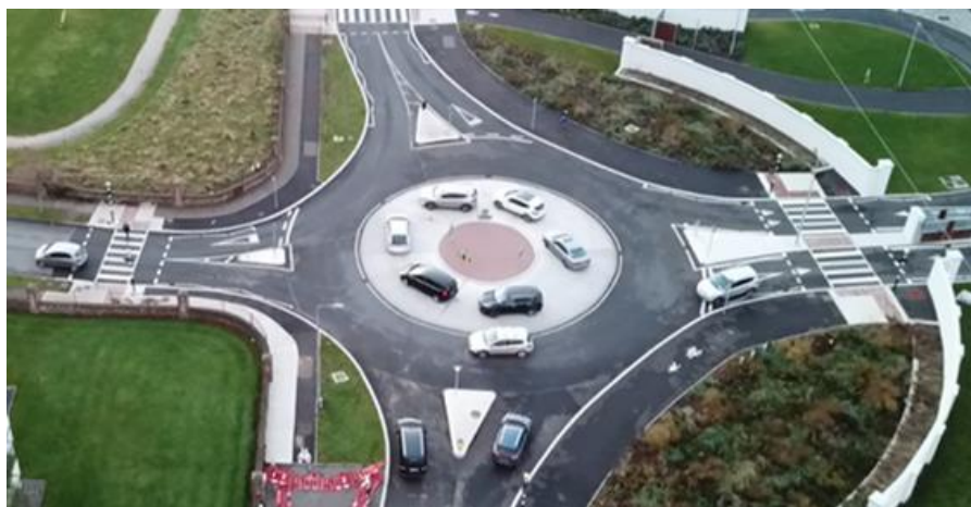
Figure 2.25 Drone Footage Showing Parents Parking on Roundabout
