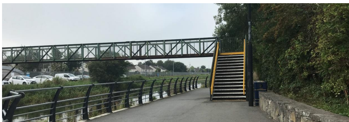
Figure 2.19 Photograph of Existing Canal Bridge
